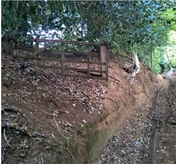
The sunken nature of the track and the rapid erosion of the sand are clearly shown here by this 'hanging gate' on Ride Lane
